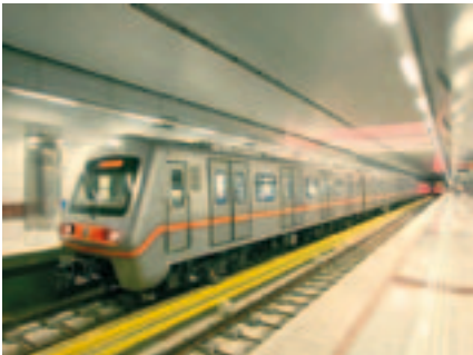
Attiko Metro stations, Athens, Greece
