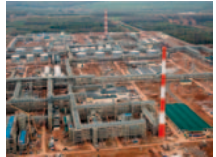
Taneco Oil Refinery, Kazan, Tatarstan
